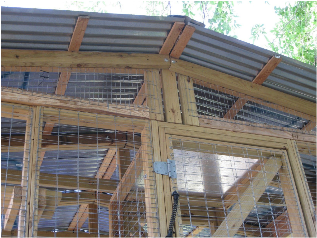
Photo showing roof modules, top screens and door module. Note plywood attached to top of airlock.
