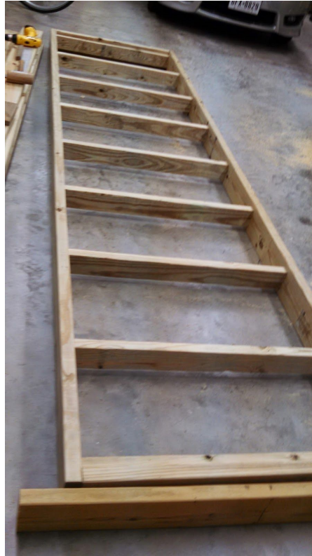
After adding stringers.
