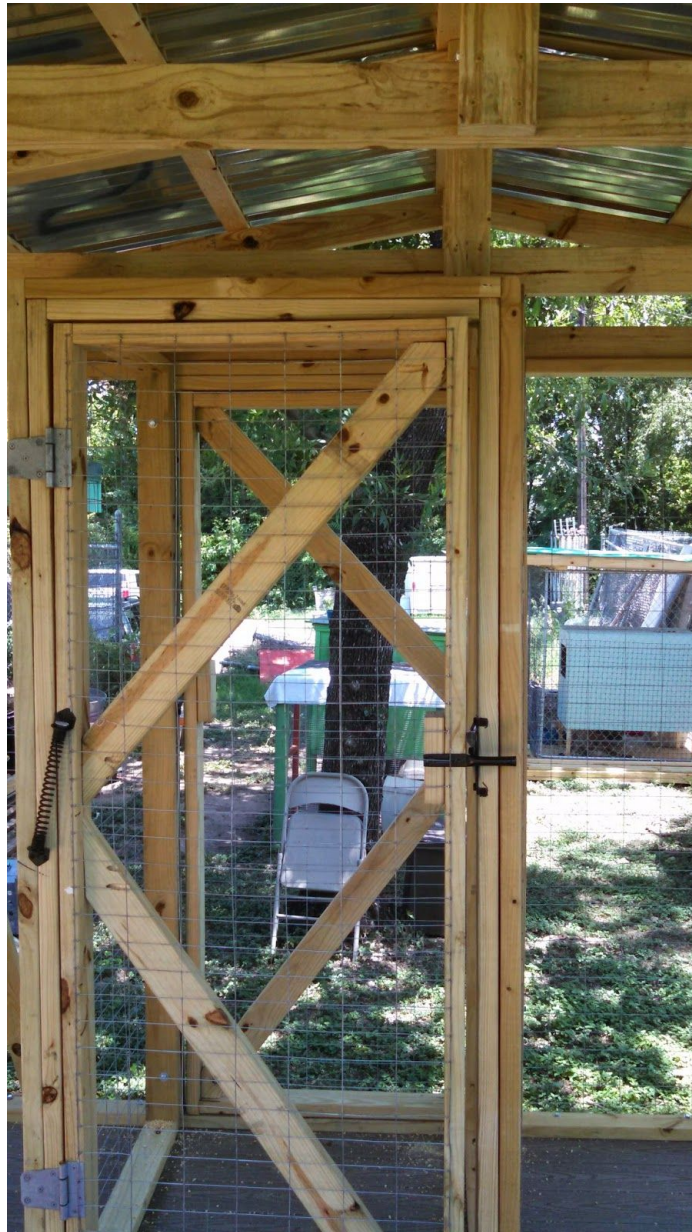
Interior photo showing inside door details and truss/roof panel details.
